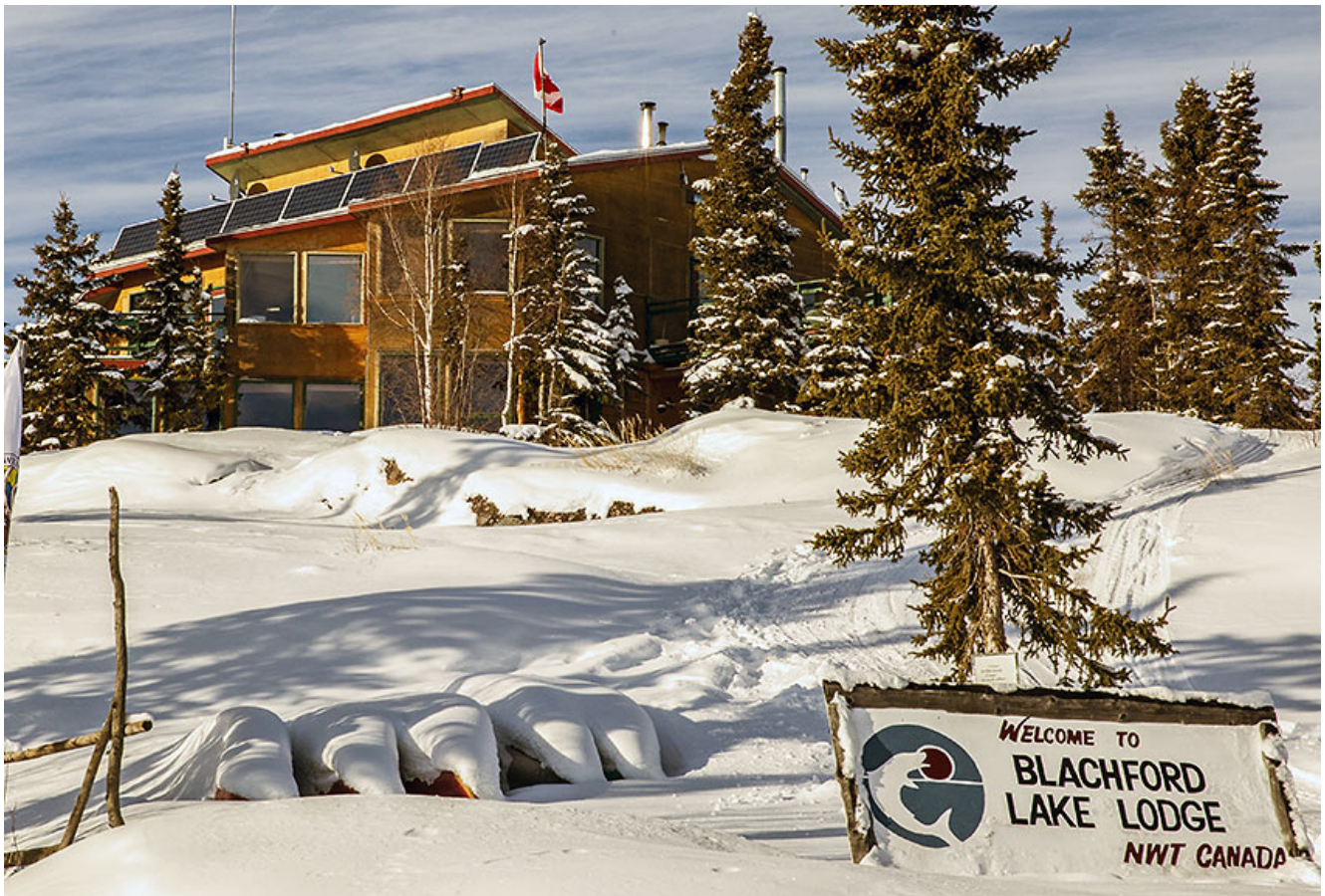
Several room additions and two rows of solar panels bring light and power to the lodge. Photo: ©Steve Haggerty/ColorWorld
