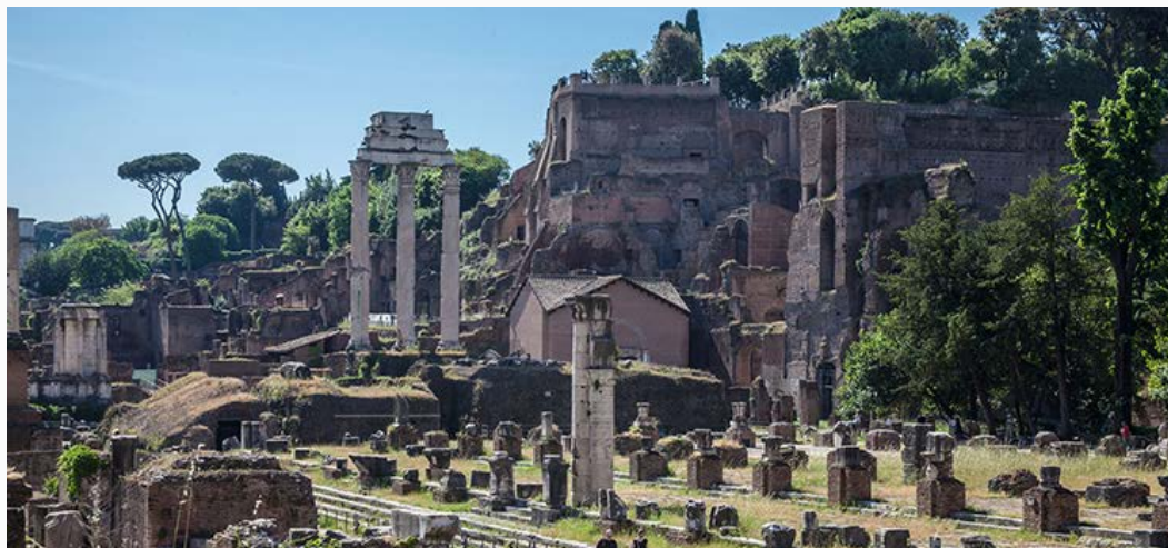
Restoration at the Roman Forum is a never-ending project that continues to reveal ancient structures. Rome, Italy. italy2015_9303--©Steve Haggerty - All Rights Reserved
