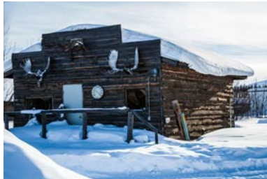
Logs: First choice for insulation against winter cold. At Coldfoot, Alaska.
